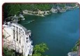
Reservoir water level measurement
